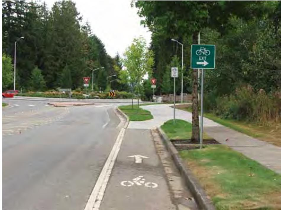
*This roundabout is designed to accommodate a bike lane.*
